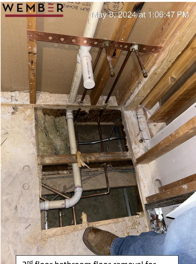
2 nd floor bathroom floor removal for making tie-ins to plumbing.
