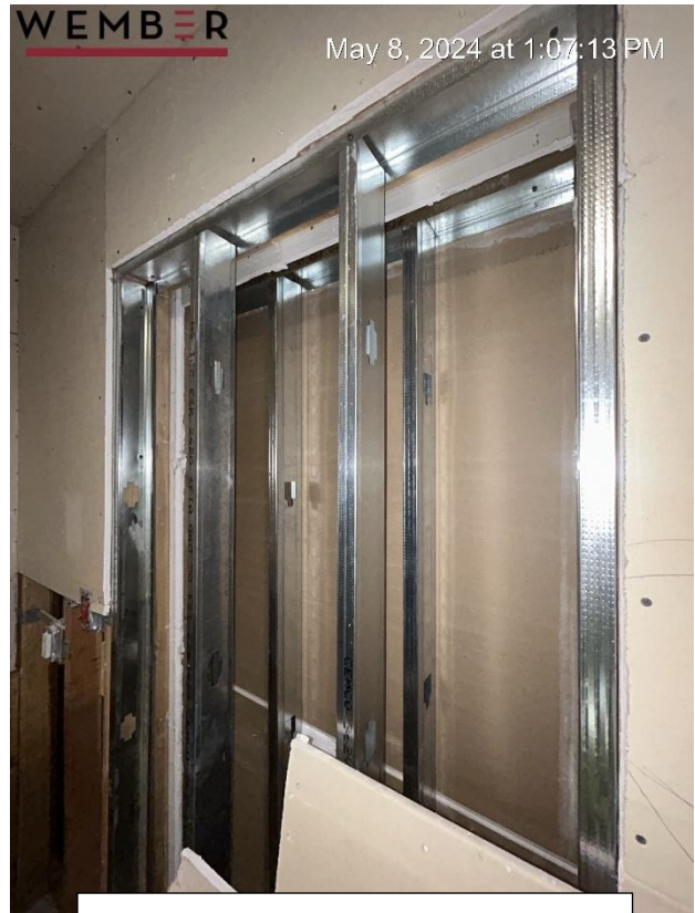
New wall framing where door to gym was demolished.
